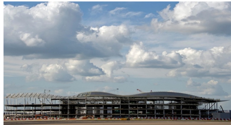
Terminal 2 site – July 2011
