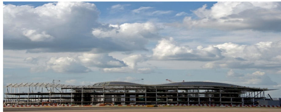
Terminal 2 site – July 2011
