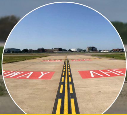
Enhanced Taxiway Centreline
