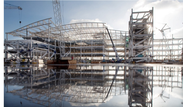
New Terminal 2 site – January 2011
