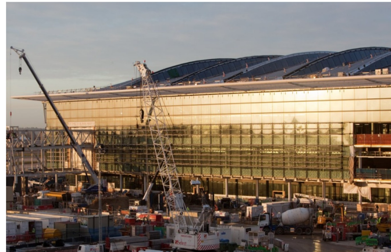
Terminal 2 site – January 2012
