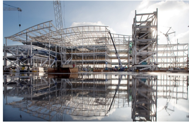
Terminal 2 site – January 2011
